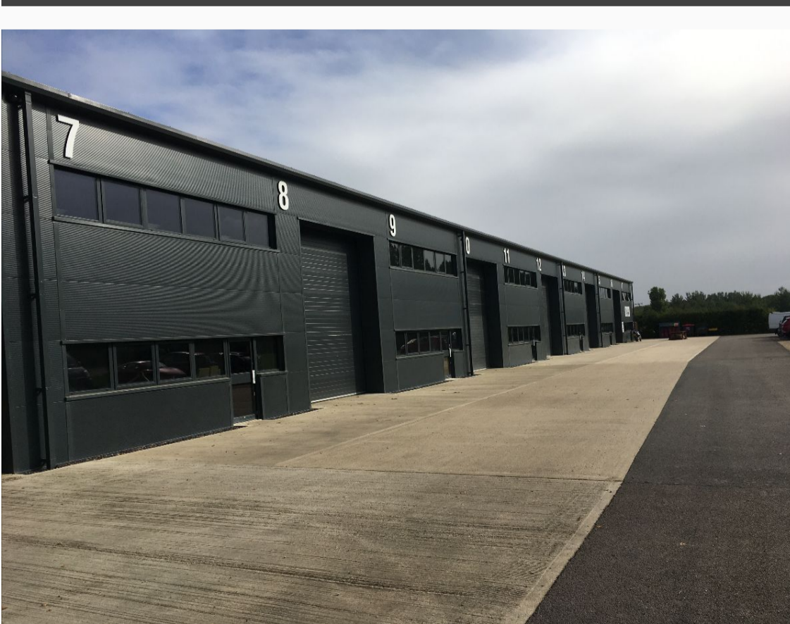
Turing Park, Norwich storage & distribution and Industrial with offices Let & Sold
